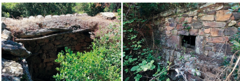
Figure 7. Left. A cellar under shelter ( 'u palmentu' ) for the fermentation of grape juice into wine at L'Elbu. Note the roof covered with earth. Right. A bread oven ( 'u furnu' ), in the wall of a stone hut. Photos © Jean-Marie Dominici.
